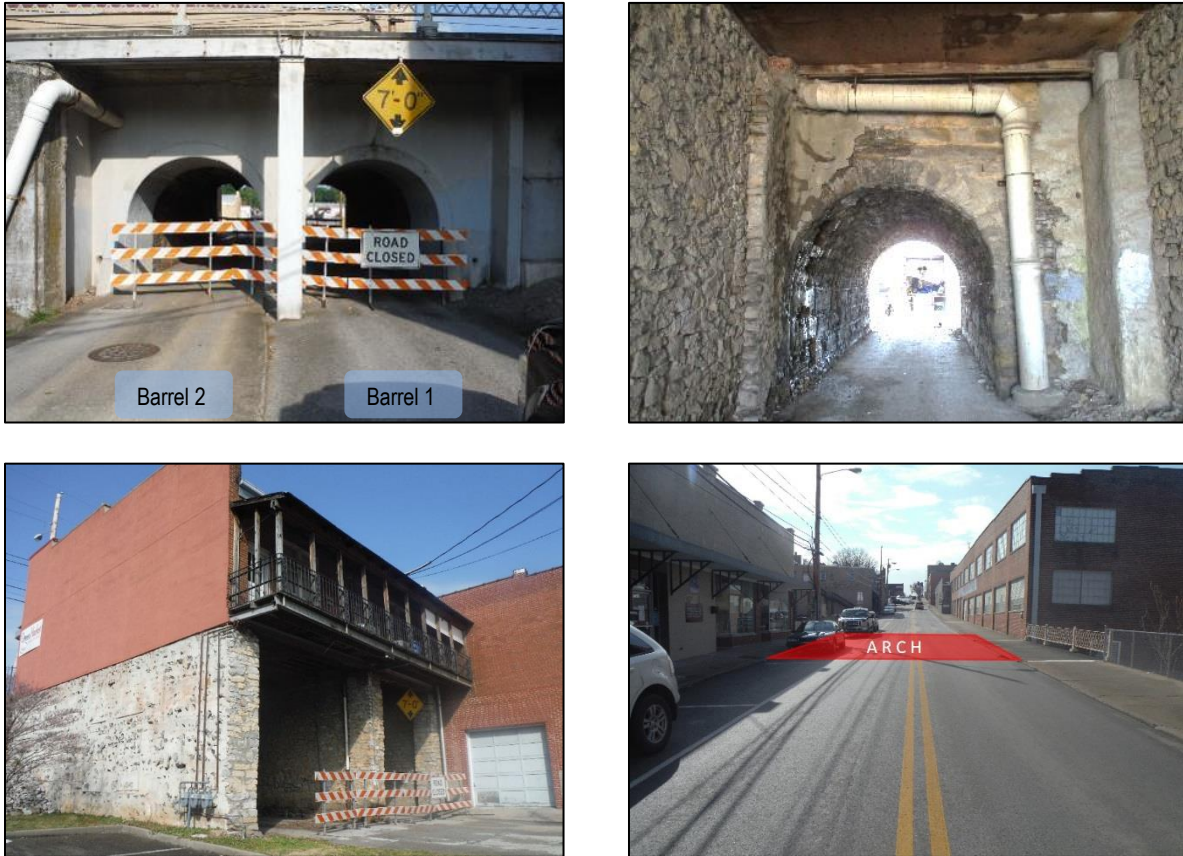
Figure 2-3: West Face of Closed Structure (Top Left); East Face Barrel 2 (Top Right); East Face and Building Walls (Bottom Left); US 31 EX Roadway on Top of Structure (Bottom Right)
